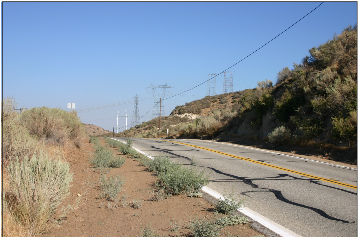
4 Elizabeth Lake Road at existing transmission line corridor crossing. Segment 2
